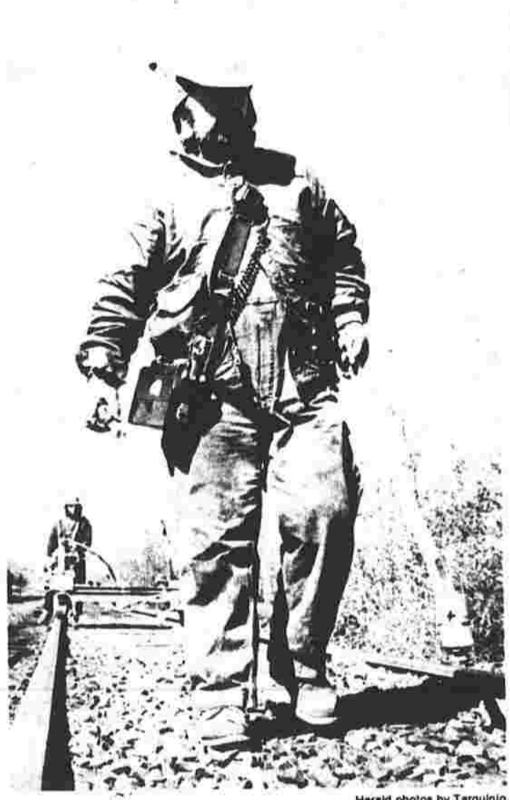
Working on the railroad
